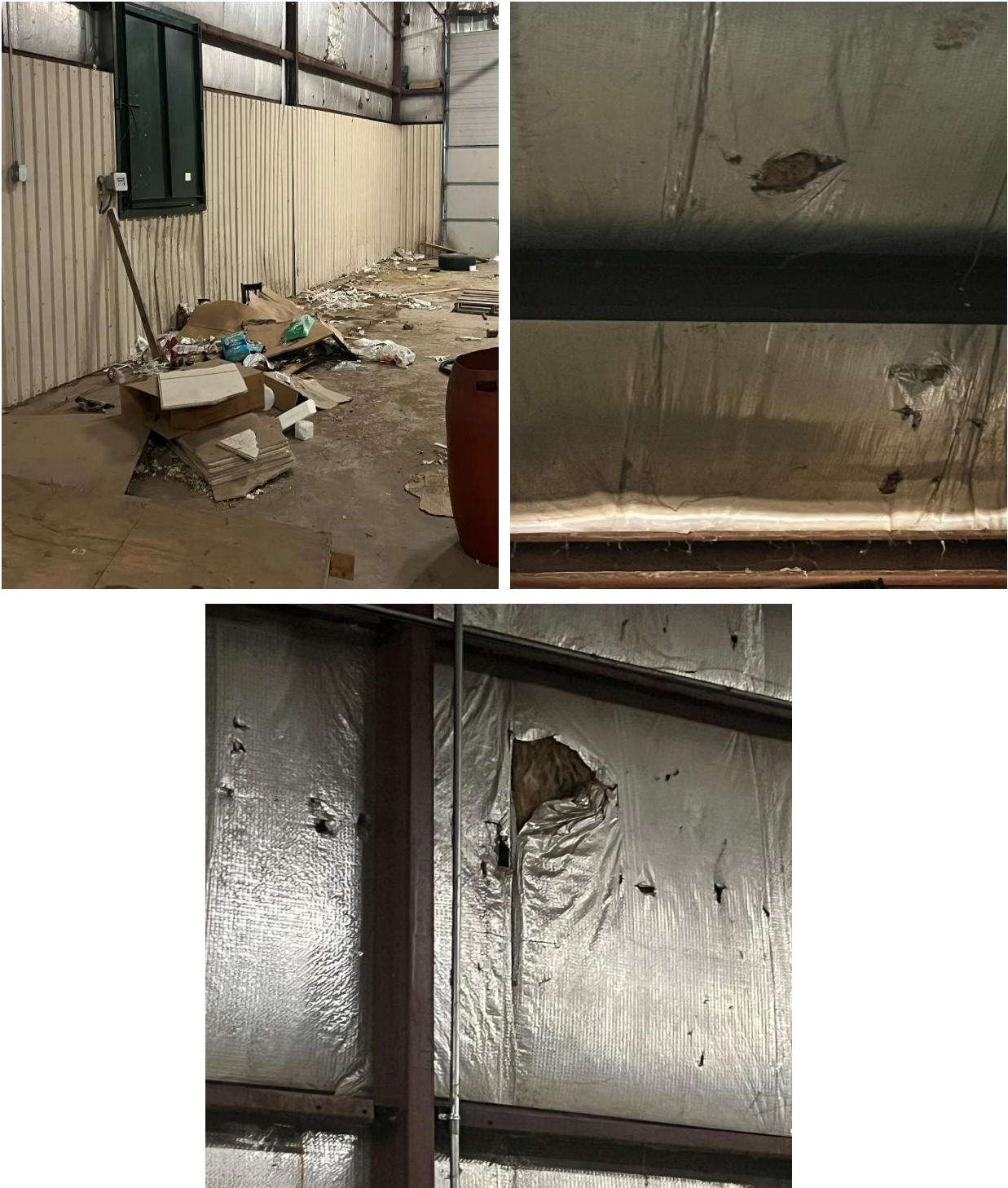
Figure 6: Degradation of Building Interior
